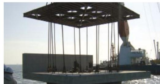
underwater weight of the pile. The load was held constant for a period of 30 minutes. No noticeable settlement of the suction piles was observed.
