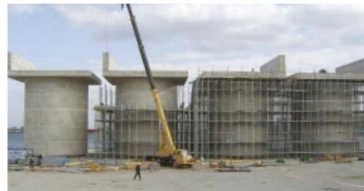
soft seafloor soil to depths where sufficient soil bearing capacity is expected. Concrete caissons are then placed on top, which resist the lateral loads caused by the wind and wave. The details of the suction pile mechanism and applications can be found in reference [1].
