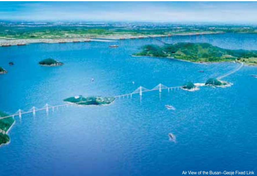
Air View of the Busan-Geoje Fixed Link
