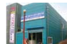
DSM Applied to Wangsong Water Treatment Plant
