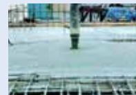
Ultra-High Flowing Concrete (FlowCrete) Placement
