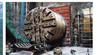
Shield TBM Tunnel (the nation's first tunnel under the Hangang (River))
