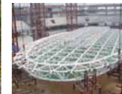
Pre-assembly of Heavyweight Structures on the Ground
