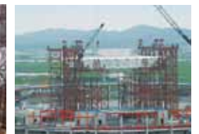
Lift-up of Structure
