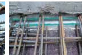
Embedded Steel Plate for Rebar splice
