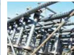
Mechanical anchorage of rebars
