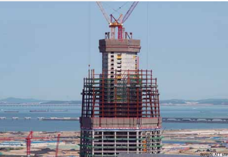
Ultra-High Flowing Concrete (FlowCrete) Placement
