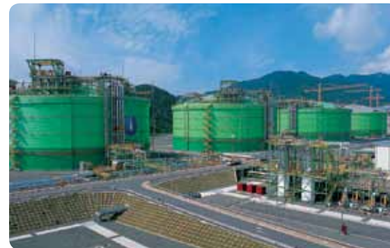
The LNG Receiving Terminal in Tongyeong
