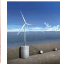
A suction pile is the basis of wind power generation
