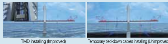
TMD installing (Improved)
