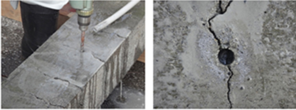
Fig. 6. Drilling of reinforced concrete cracks
